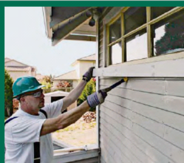
A small, thin prybar is indispensable for removing delicate trim from both the interior and exterior of a house during deconstruction.
